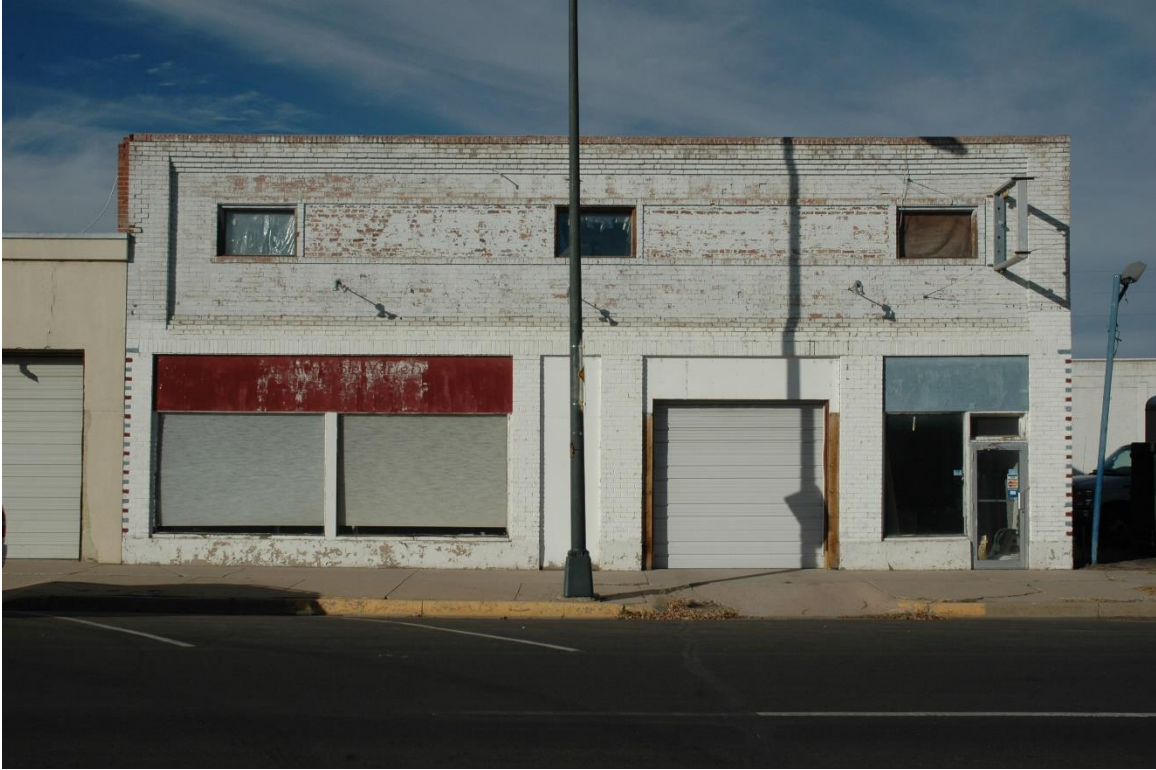
CD 1, Image 158, View to north of 723 - façade (south)
