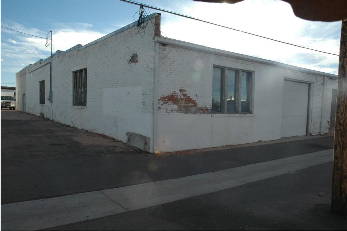
CD 1, Image 162, View to SW of 715 – east and north sides
