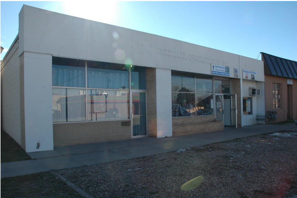
CD 2, Image 16, View to SW of façade (north)
