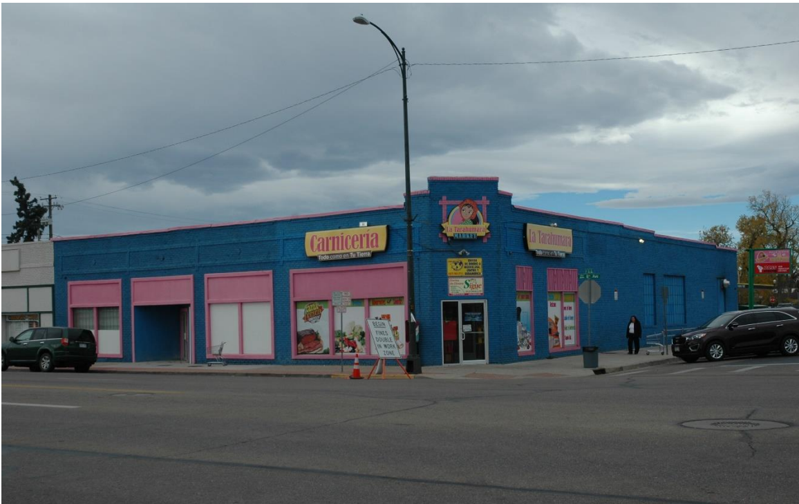
CD 1, Image 15, View to SW of façade (east) and of north side
