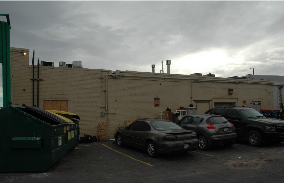
CD 1, Image 18, View to ESE of rear (west)
