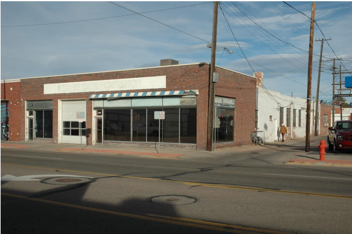
CD 1, Image 178, View to NE of façade (west) and south side
