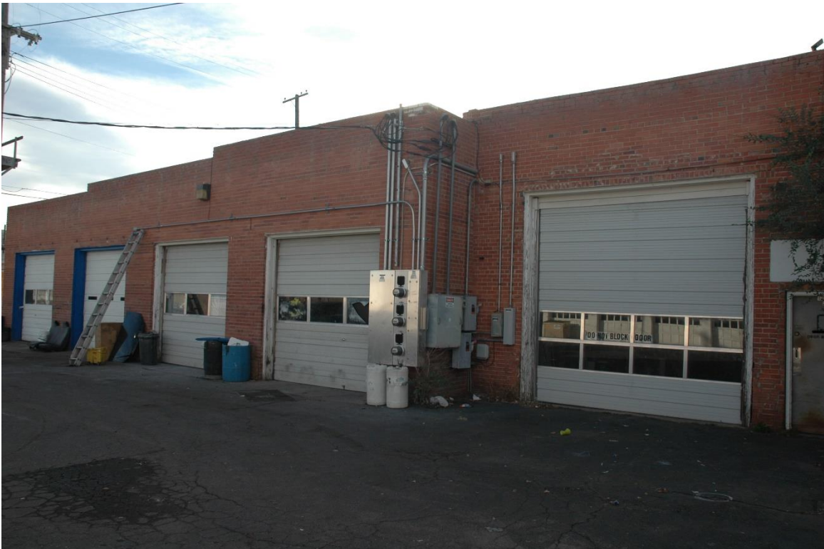
CD 1, Image 181, View to WSW of rear (east)
