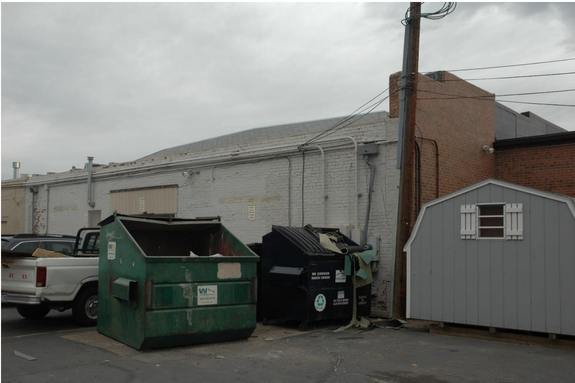
CD 1, Image 23, View to NE of rear (west)
