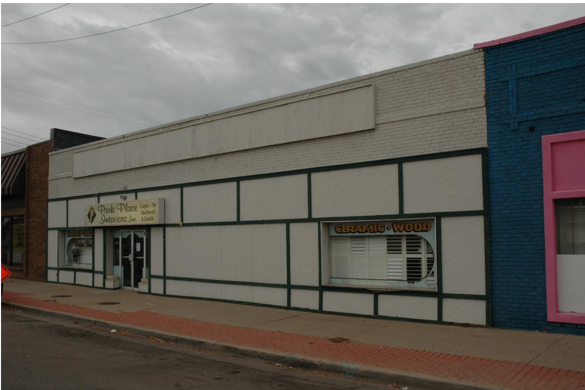
CD 1, Image 21, View to SW of façade (east)
