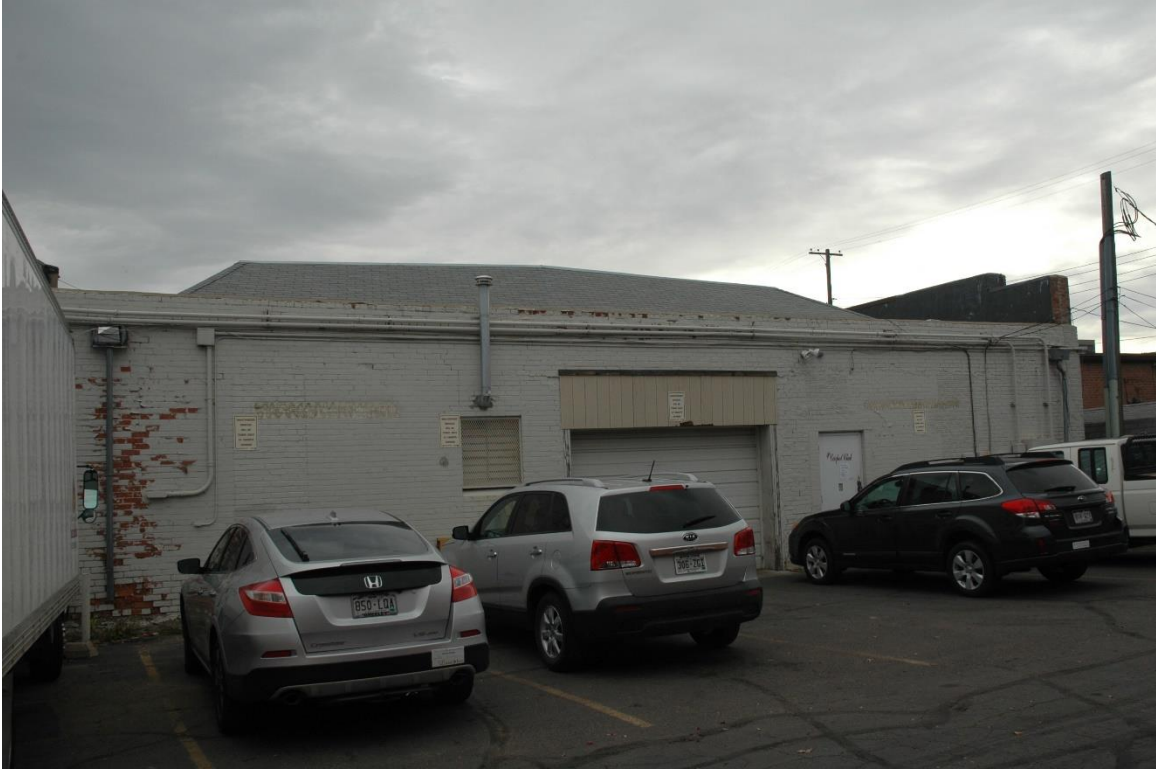
CD 1, Image 22, View to ESE of rear (west)
