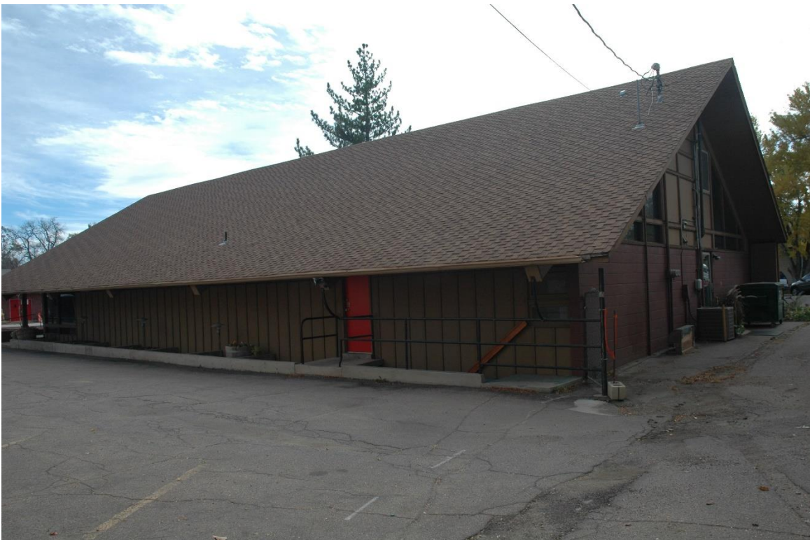
CD 1, Image 82, View to SE of north side and rear (west)
