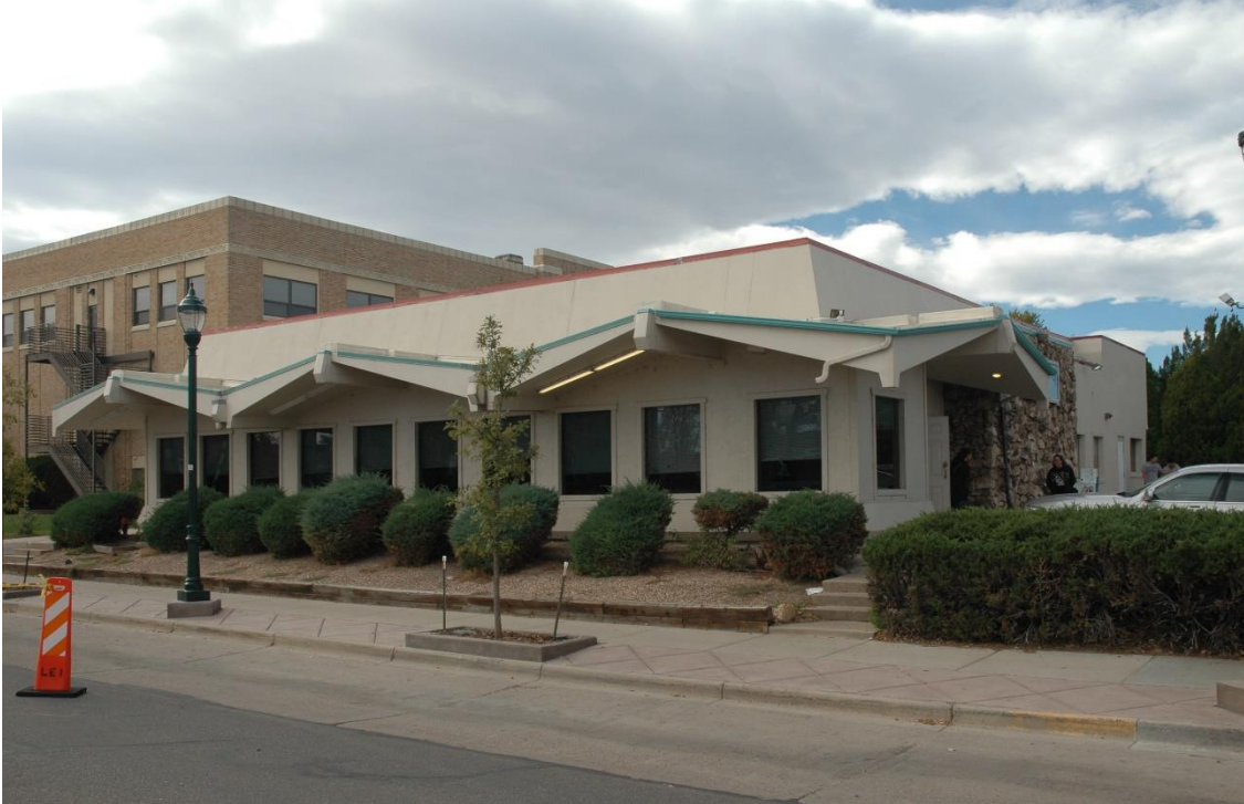
CD 1, Image 88 View to SW of east and north sides
