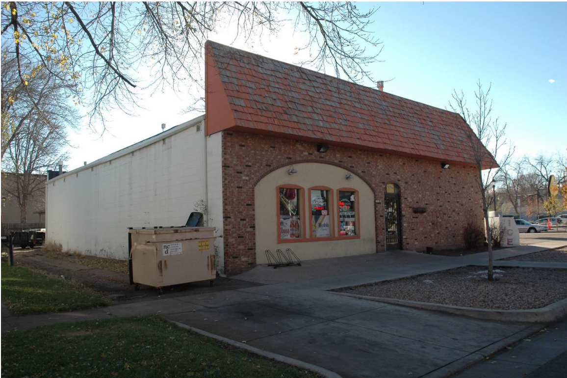
CD 2, Image 34, View to SW of east side and of front of building facing 15 th Street to the north
