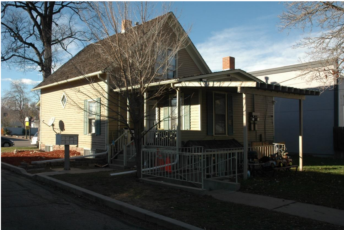
CD 2, Image 41, View to NW of south side and rear (east)
