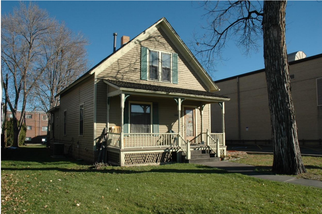
CD 2, Image 39, View to SE of façade (west) and north side
