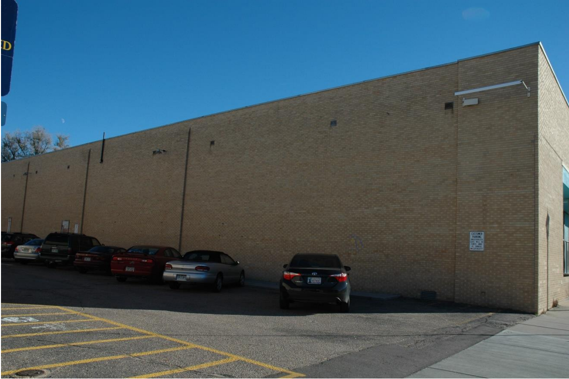
CD 2, Image 48, View to SE of north side
