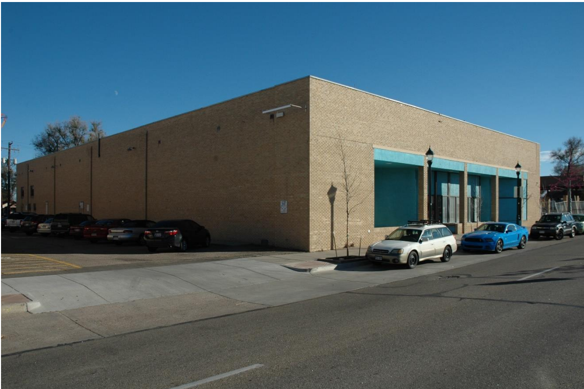
CD 2, Image 49, View to SE of north side and façade (west)
