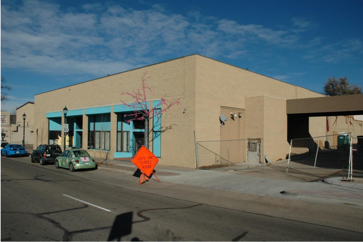
CD 2, Image 50, View to NE of façade (west) and south side
