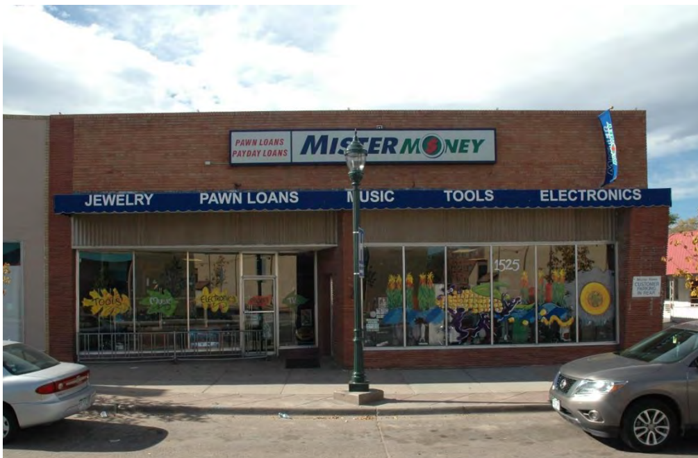
Pioneer Saving Stamp Redemption Center building, 1525 8 th Avenue (5WL.7850) Built 1953 Photo by Carl McWilliams, September 2015
