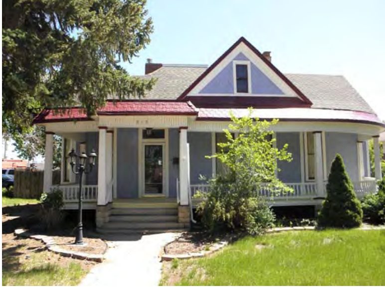
Sterling House, 818 12 th Street, 6 June 2014
