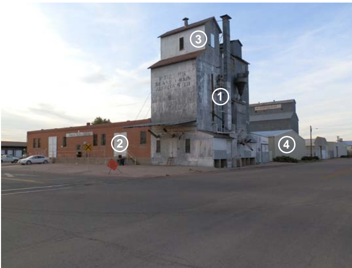
Grain Elevator - 601 10th St. - L. Schaffer, 09/24/2011
