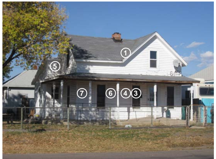
Folk Victorian House - 531 9th St., ca. 1880 - Greeley Historic Preservation Office, Colorado State University interns, 10/19/2010
