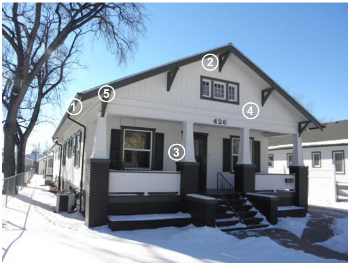
Craftsman House - 426 11th St., ca. 1926 - Greeley Historic Preservation Office, Colorado State University interns, 1/13/2011
