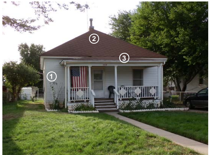
Hipped-Roof Box House - 1519 3rd Ave., ca. 1900 - L. Schaffer, 9/24/2011
