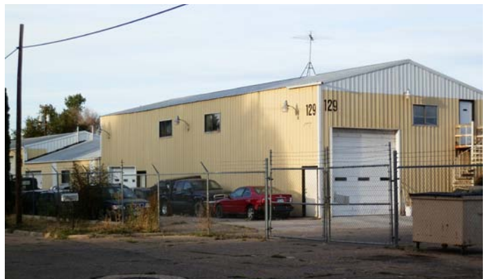
Warehouse/Storage - 129 12th St. - L. Schaffer, 09/24/2011
