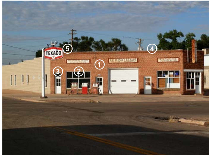
Texaco Station - 531 8th St. - L. Schaffer, 09/16/2011
