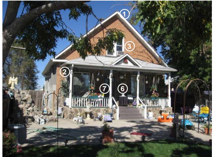
Folk Victorian House - 417 6th St., ca. 1890 - Greeley Historic Preservation Office, Colorado State University interns, 9/28/2010
