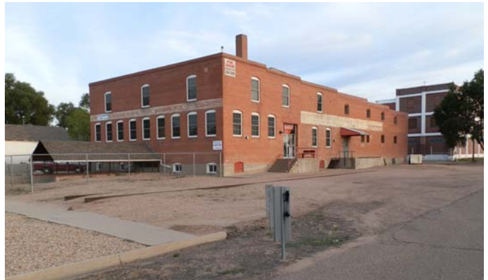
Industrial - 6th Ave. - L. Schaffer, 09/24/2011
