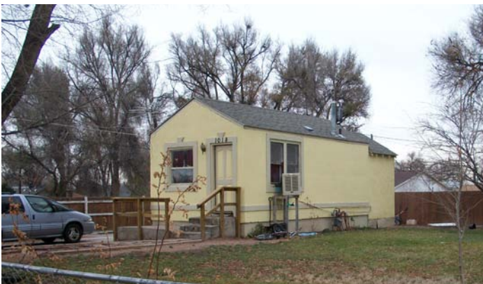
Shotgun - 1018 3rd Ave. - Greeley Historic Preservation Office, Colorado State University interns, 11/18/2010
