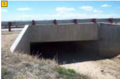
Greeley-Loveland Canal crossing at 77th Ave.
