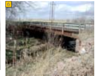
6 Existing bridge at 83rd Ave. Height and width will not accommodate trail underpass. Future road construction plans should accommodate trail on north side of drainage.
