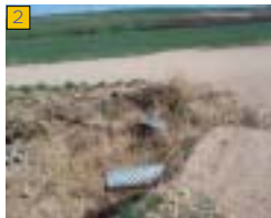
2 Small culvert passes drainage under 95th Ave.
