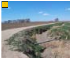
1 Trail west of 95th Ave. runs along ditch rider road.
