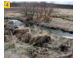
Existing drainage channel and wetlands southeast of detention pond have been damaged extensively by construction, but will be a great trail amenity if restored.
