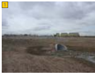
Existing condition of drainage crossing at 18th St.
