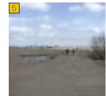
Dam and detention pond at Boomerang Ranch. Wetlands and existing drainage channel on the right. Development plans do not show a trail along north side of detention pond, so trail must cross spillway.
