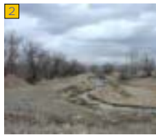
Existing drainage just east of 71st Ave. To preserve existing wildlife habitat and vegetation, the trail is located on the north edge (behind) of the trees, on the left side of the photo.
