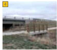
Existing Sheep Draw pedestrian bridge south of 10th St.
