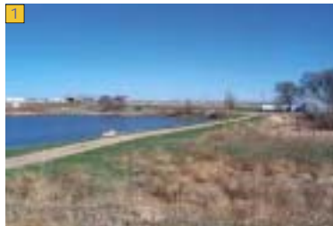
1 Looking north along edge of dam from trail alignment.
