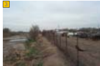
Some areas of the existing salvage yards have eroded slopes, and no room exists for a trail unless fill and bank stabilization measures are implemented.
