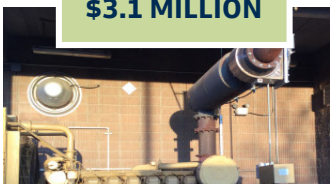
Wastewater Treatment & Reclamation Facility (WTRF) Generator Replacement
