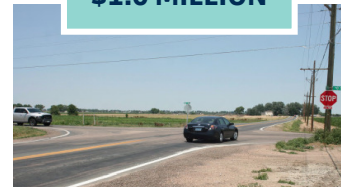
Intersection Improvements at 35th Avenue & "O" Street Roundabout
