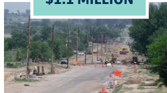
35th Avenue Road Widening: 4th Street to "F" Street
