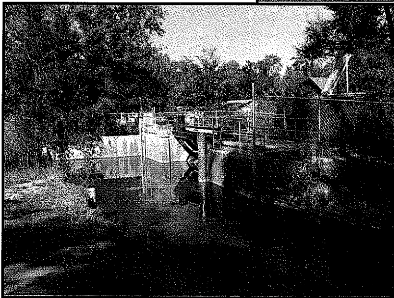
Clarkson Spill Structure on the Greeley No. 3 Ditch
