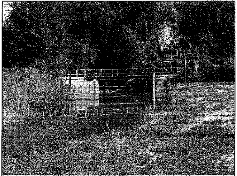
Figure 2.4 Clarkson Spill Structure.
